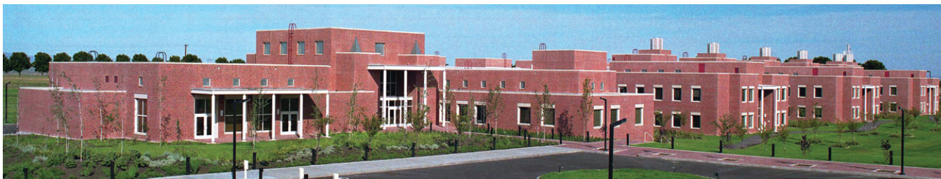
Photo 1: Significant energy costs were avoided at EMSL, a 200,000 ft 2 national scientific user facility for research, despite energy-intensive equipment such as supercomputers.
